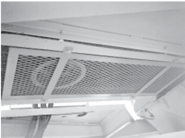
*Properly installed belt guard*
