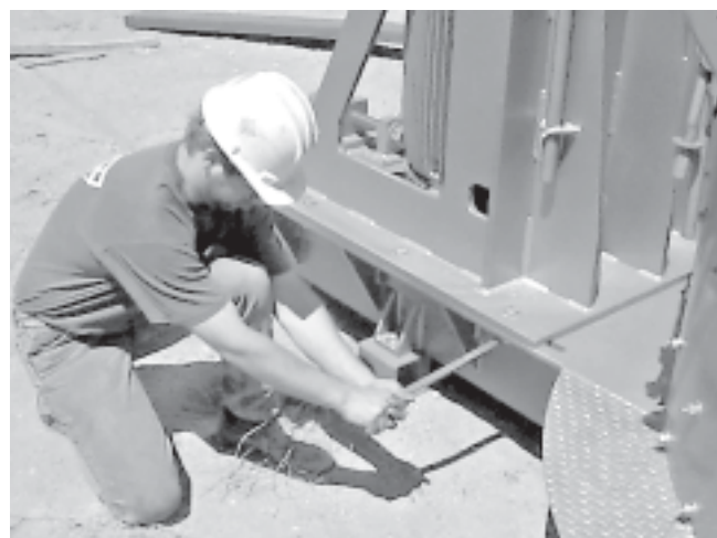
Loosening the motor mount bolts
