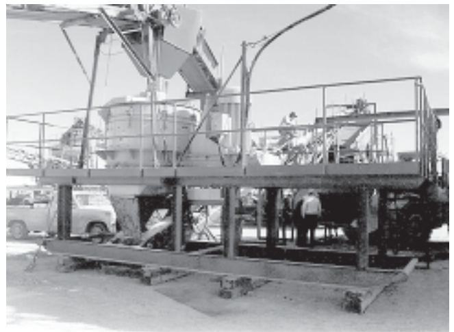
Skid mounted unit
